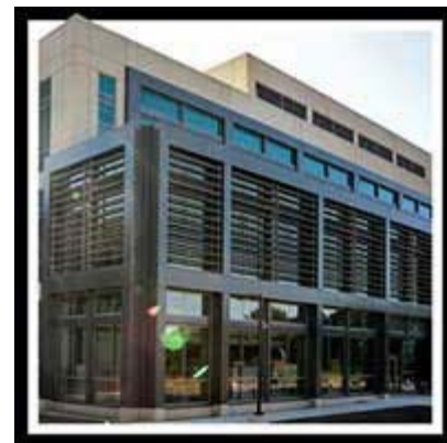
Science and Engineering Laboratory Building
