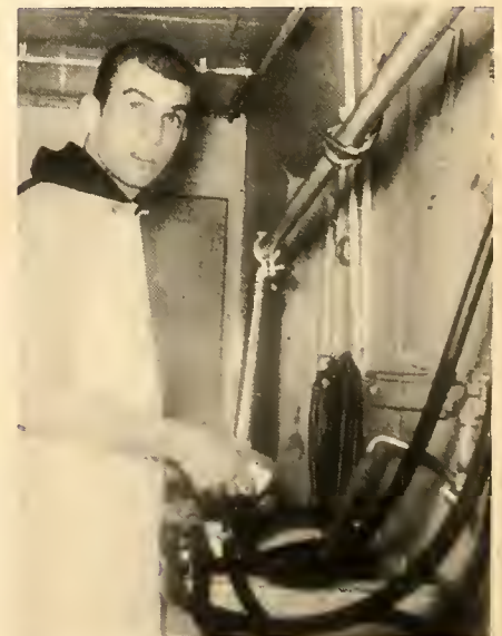
Helmut had to increase the size of the milkhouse to install the new bulk tank.
