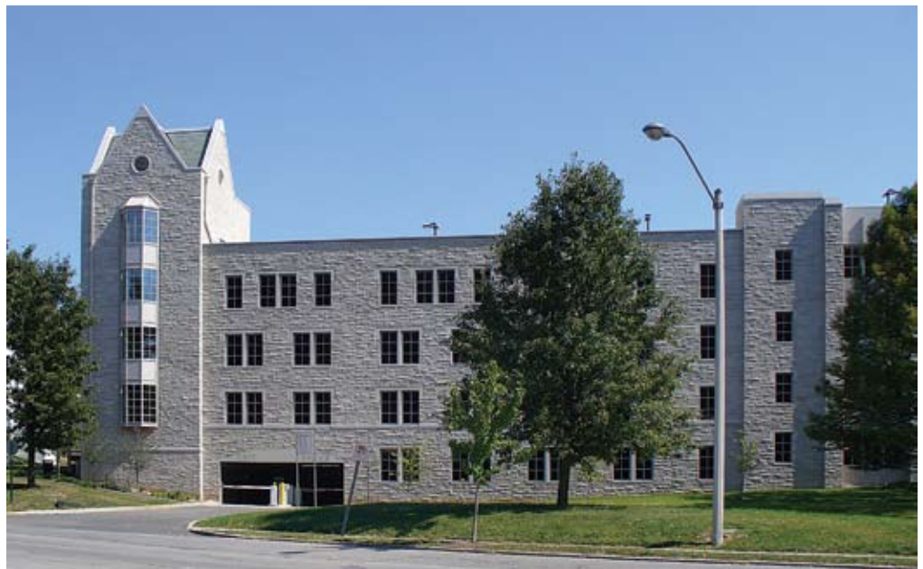
Henderson Garage and Parking Operations, IUB
