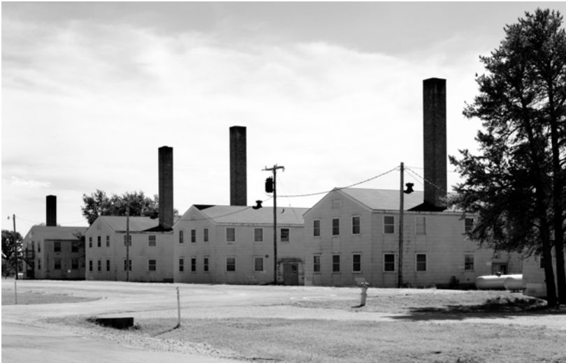
Barracks at Camp McCoy. Library of Congress, Historic American Buildings Survey/Historic American Engineering Record (HABS, WIS,41-SPAR.V1-21).
