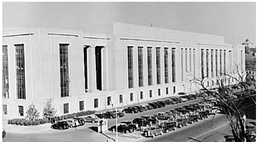
Social Security Building, Washington, D.C. Library of Congress, Prints and Photographs Division (LC-USE6-D-002115).
